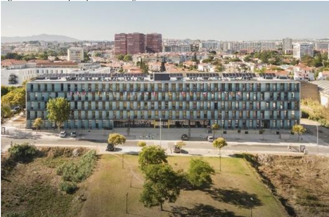
Figura 03 – Fachada principal do Co-living Carcavelos.
